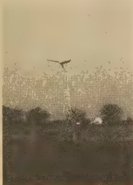
BOTH THESE WINDMILLS USE OCTAHEDRON TOWERS
